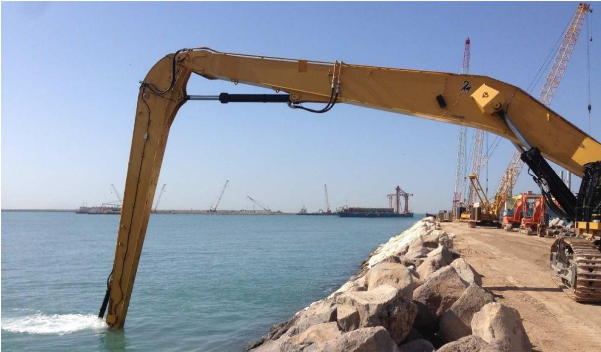
**Figure 5. Customized 29 m (95 ft.) long-reach excavator at work in breakwater construction.**
