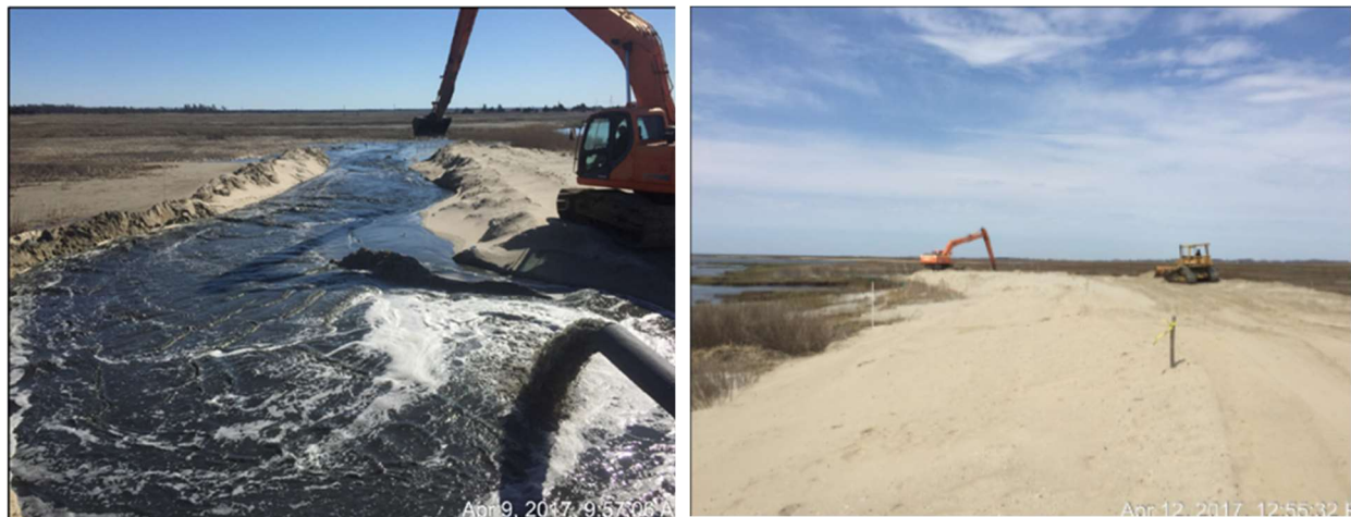
Figure 9. Settling trench for dune construction (a) and shaping of dune with grade stake in foreground (b).
