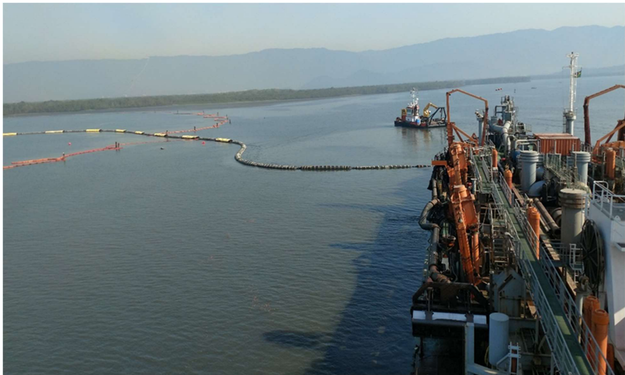
Figure 7. TSHD performing pumping through HDPE piping to fill the CAD.
