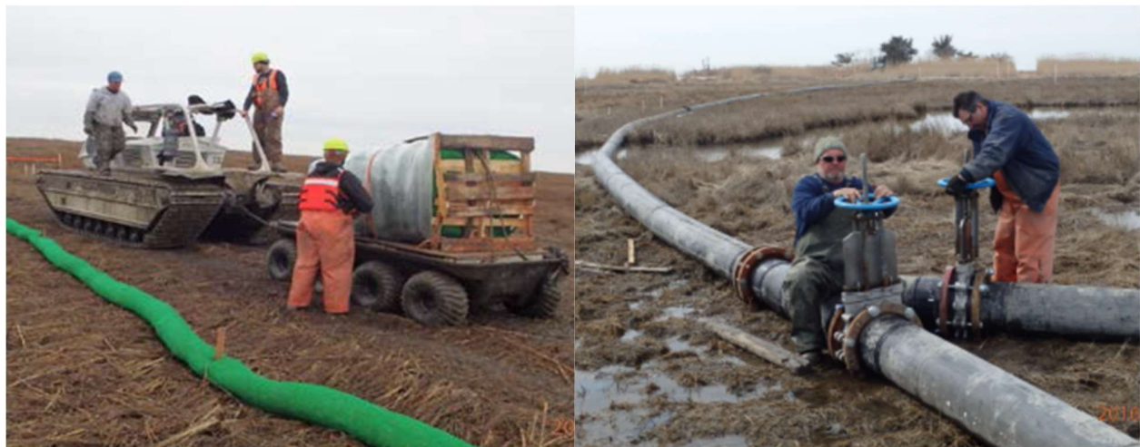
Figure 6. Perimeter containment installation (a) and contractor utilized distribution array (b)
