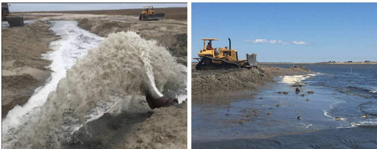
Figure 10. Settling trench for beach placement (a) and bulldozer grading sand to beach template (b).
