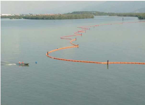
Silt curtain around the CAD
