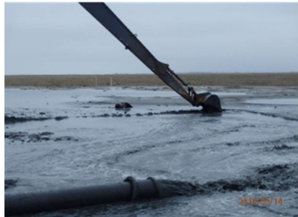
Figure 8. Dredged slurry being pumped on marsh (a); distributed with long reach excavator (b)
