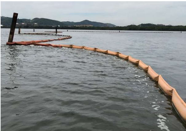
Silt curtain details installation
