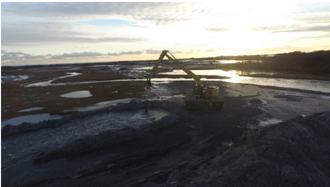
Figure 4 Discharge control in the designated marsh area
