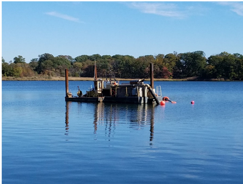
Figure 2. Barracuda 12-inch cutterhead pipeline dredge working in Shark River Bay.
