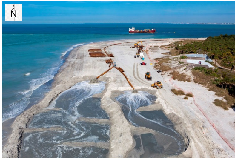
Figure 4. Traditional beach placement at northern end of Egmont Key, FL, 26 December 2014. Photo courtesy of GLDD.
