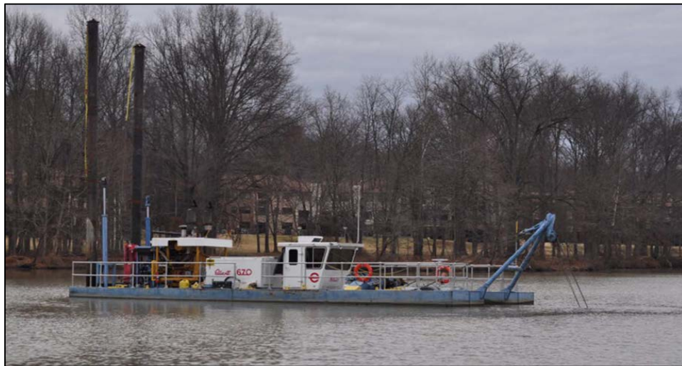
Figure 6. Lake Kittamaqundi Dredging
