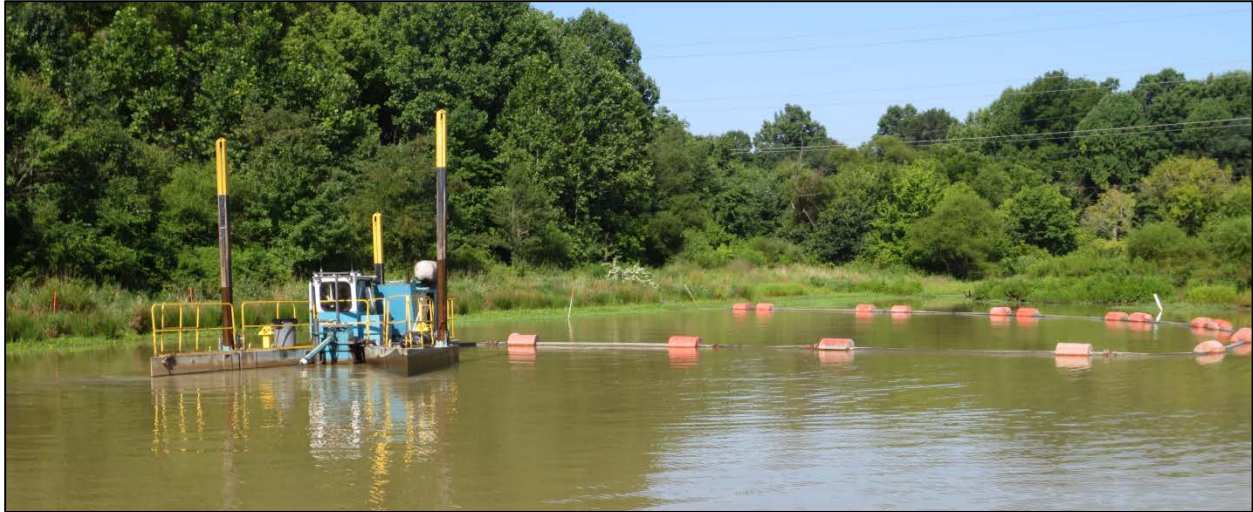
Figure 8. Hydraulic Dredging Operations
