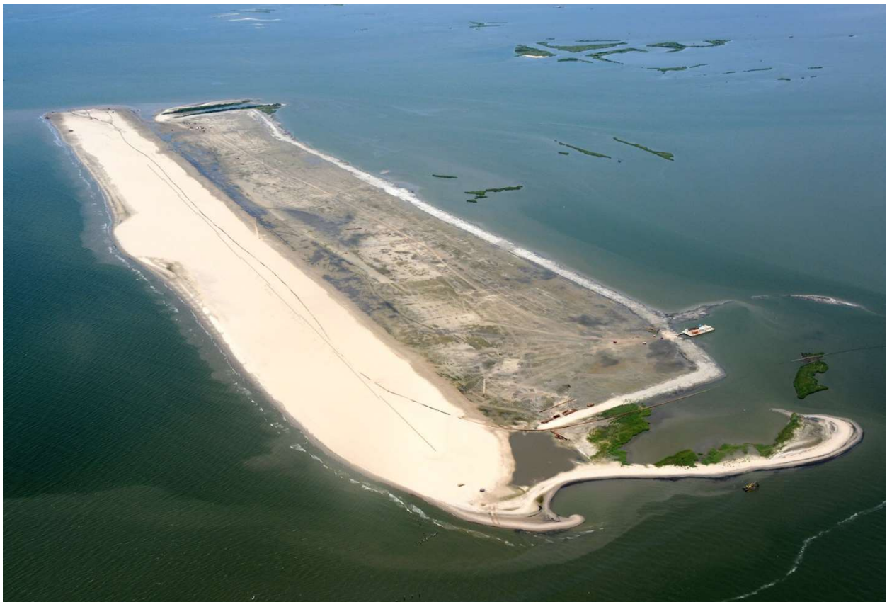
Shell Island East Barrier Island Restoration (photo courtesy of Great Lakes Dredge & Dock Company, LLC)
