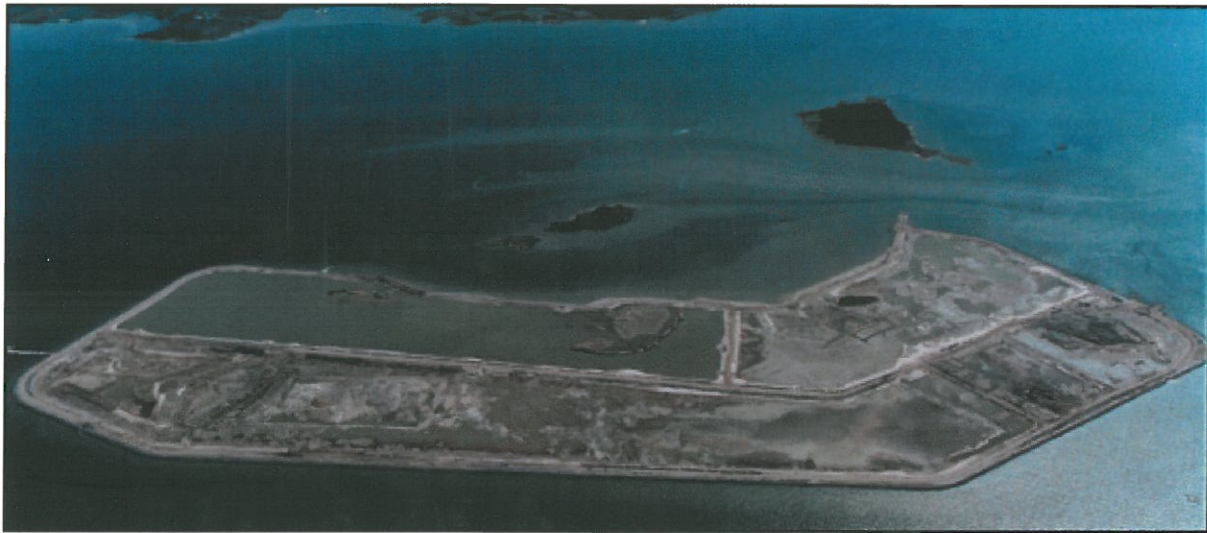
Popular Island Restoration Project, Chesapeake Bay, Maryland
