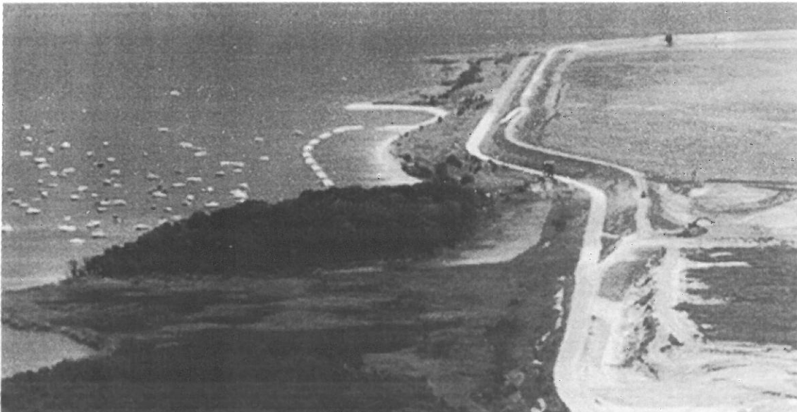
Figure 6. West side of Hart-Miller Island during the summer boating season. Recreational beach protected by segmented breakwaters shown in center of picture. ( L. D. Heath, MES )
