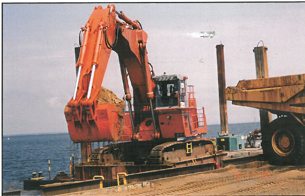
Mechanical Excavator (courtesy of Gahagan & Bryant Associates, Inc.)
