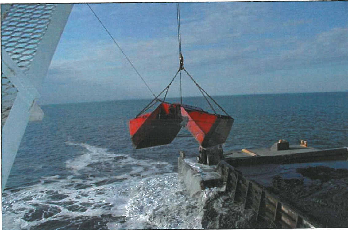
Cable-Arm Clamshell Bucket
