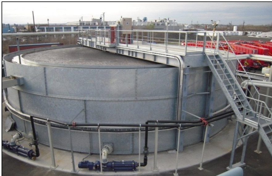
Figure 12. Gravity thickener
