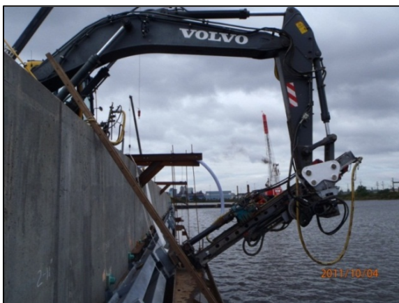
Figure 2. Tieback installation
