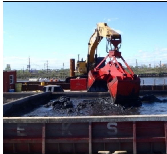
Figure 7. Dredge placing sediment into barge
