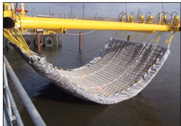
Figure 3. Setting concrete mattress into place
