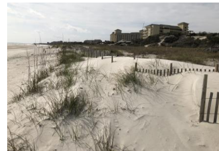
Beach and Dune Construction
