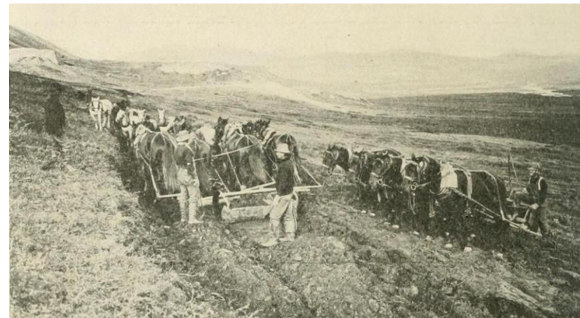
Miocene Ditch construction, Nome River, AK, 1901-03
