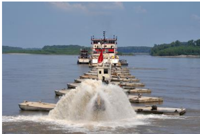
Sediment “Recharge” via Dredging
