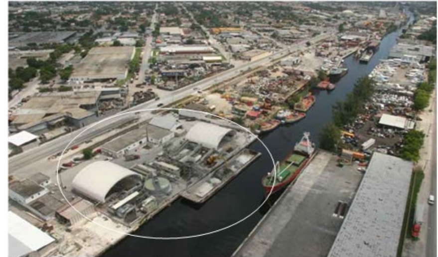
Figure 1.2 Photograph of Boskalis-Dolman physical separation system, Miami River, FL (Courtesy Bastiaan Lammers, Boskalis Dolman).
