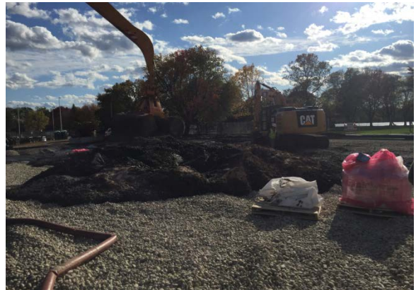
Photo 6: Sediment stabilization using Calciment
