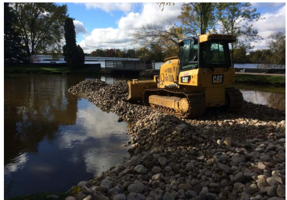
Photo 4: Construction of temporary causeway in the Pond
