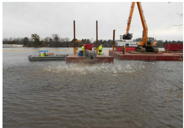
Photo 18: Armor layer placement in the River
