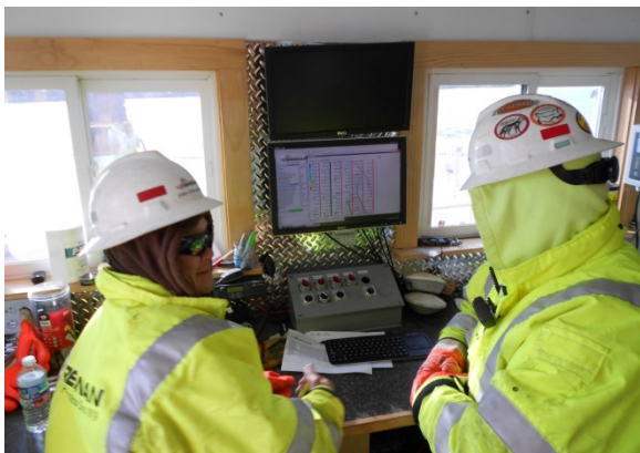
Photo 17: BCS™ control room
