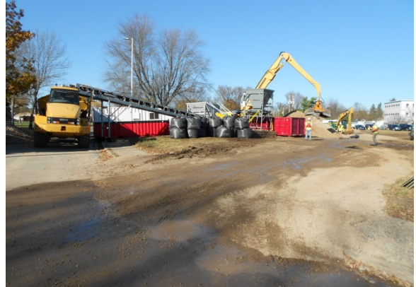
Photo 14: Adsorptive cap (GAC and sand) mixing system
