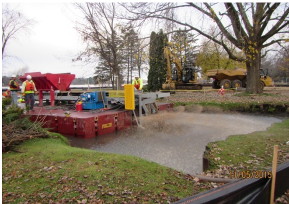
Photo 15: Adsorptive cap placement in the Pond using the BCS™
