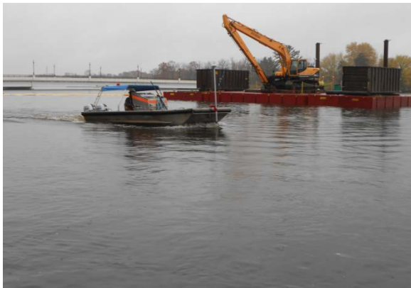
Photo 11: Hydrographic surveying River dredge area
