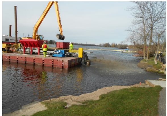
Photo 16: Adsorptive cap placement in the River using the BCS™
