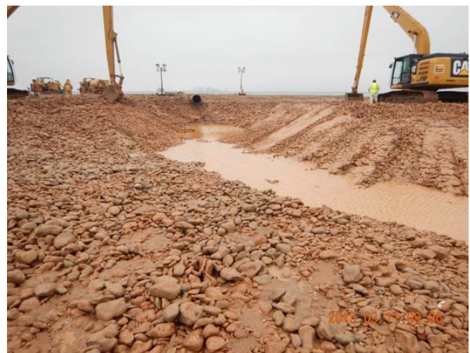
Equipment shaping clay balls to raise the levees at PA 15
