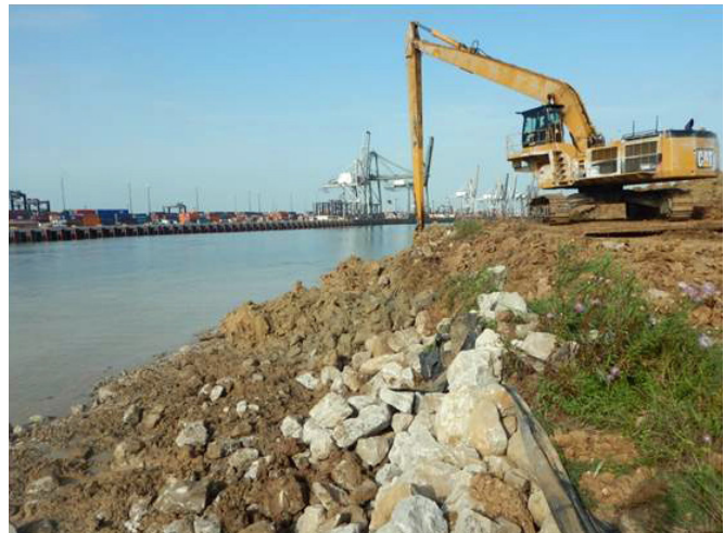
Shore protection being redistributed to accommodate channel modifications
