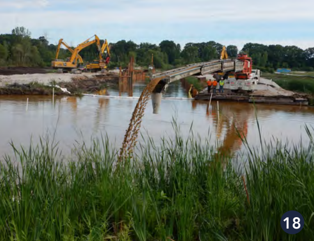
14. Portland cement addition as last step in dewatering of sediments
