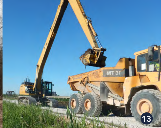
12. In-situ mixing to stabilize hazardous sediment 13. Multiple dredging methods utilized and constructed haul roads for site access
