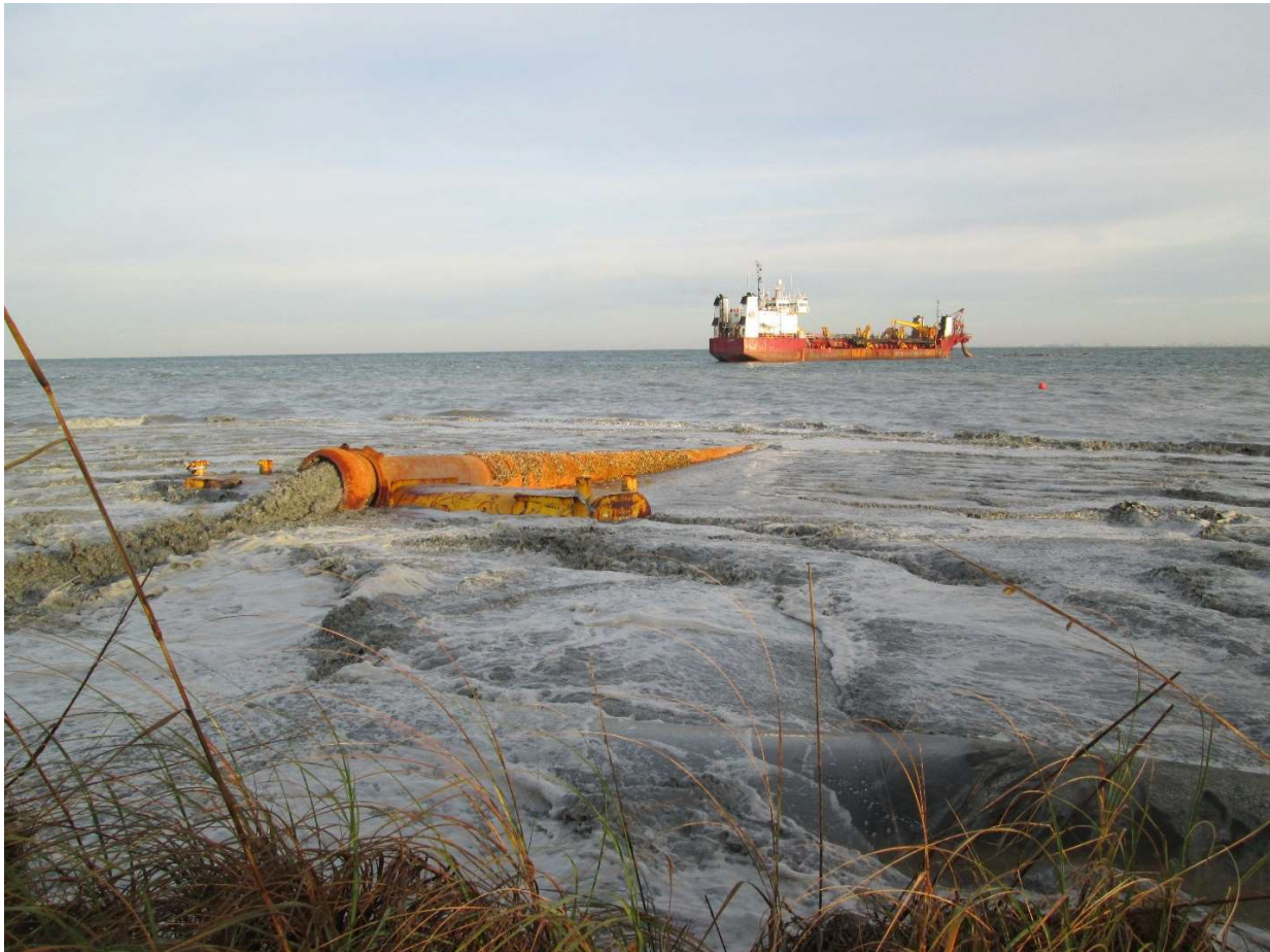
Discharge of navigation dredged material from the Dodge Island for beneficial use on Egmont Key, Florida. Photo courtesy of Coraggio Maglio, US Army Corps of Engineers.
