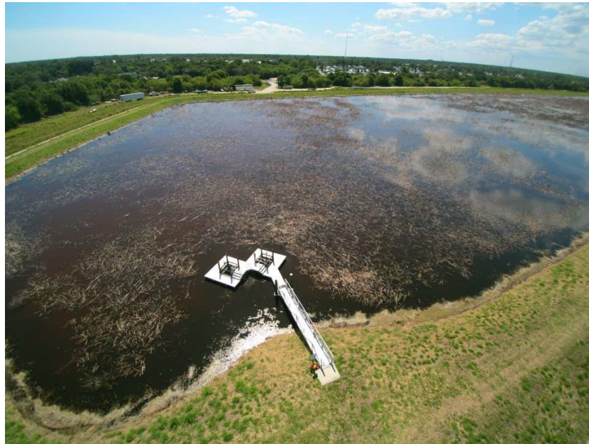
Figure 3. Dredged Material Management Area IR-2 and water control weirs 14 May 2015. Photo credit Cavache Inc.
