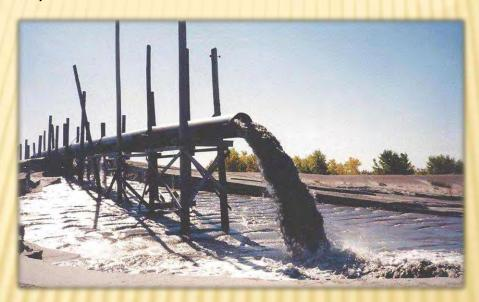
The dredge will typically remove 10 feet of sediment from the canal. Approximately 1.5 to 1.6 million cubic yards of sand is taken from the canal each year.
