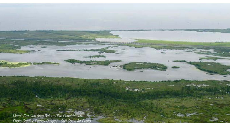
RM WHITE Pumping 6.15 Million Cubic Yards of material ashore into 3 Marsh Creation Area Cells as part of the LaBranche Marsh Creation Project. Photo Credits: Patrick Quigley - Gulf Coast Air Photo
