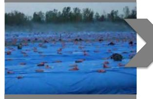
Change required handling of hundreds of sand bags and decreased footing on wet, slippery, uneven surfaces Worked with Geotubes manufacturer to install pre-covered tarps before shipment, eliminating sand bags
