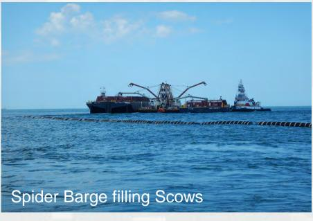
Requirement: Deepen the Entrance Channel from -44' MLLW to -49' MLLW and extend the channel 7.1 miles seaward; removing approximately 11 million cubic yards of new work material
