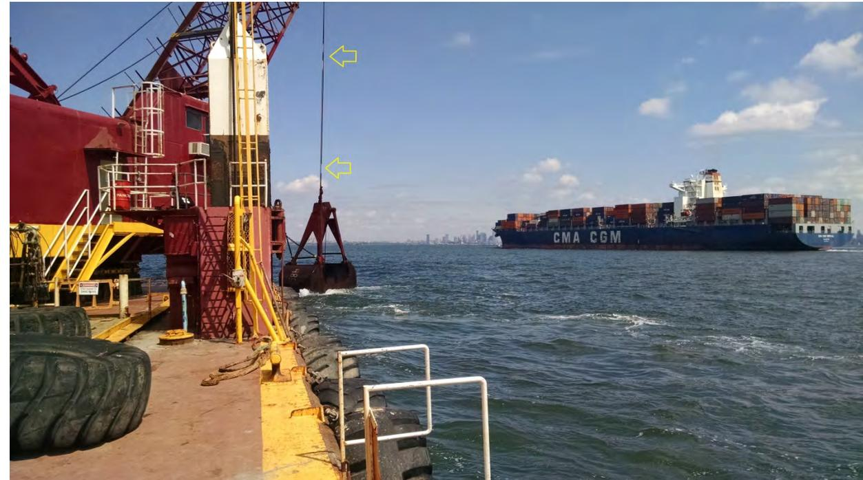
Figure 8. Dredging Operation in Progress (yellow arrows indicate cable markings for depth control and dredge bucket open/close check)
