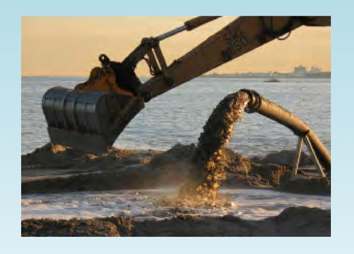
• Dredging is the form of excavation carried out underwater or partially underwater, in shallow waters or ocean waters. It keeps waterways and ports navigable, and assists coastal protection, land reclamation and coastal redevelopment, by gathering up bottom sediments and transporting it elsewhere. Dredging is a four-part process: loosening the material, bringing the material to the surface (together extraction), transportation and disposal.
