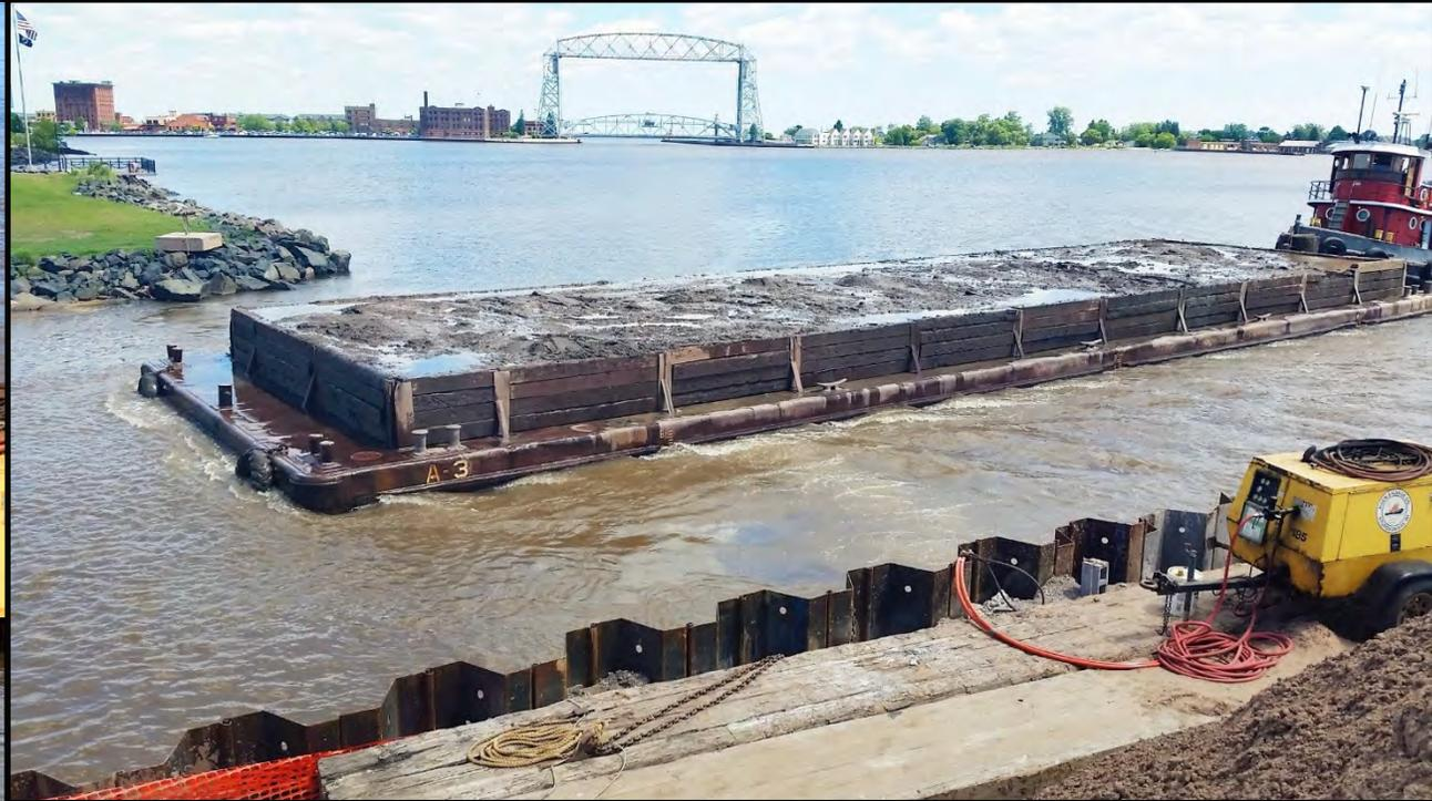
**A Bubble Curtain was used to contain suspended solids and allow for frequent barge transport**
