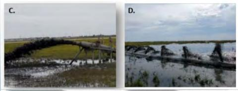
Placement at (A) Gull and (B) Sturgeon Island. (C) Dredged slurry being pumped on southern Gull Island. (D) Innovative sediment distribution pipe being utilized as part off the Sturgeon Island placement.
