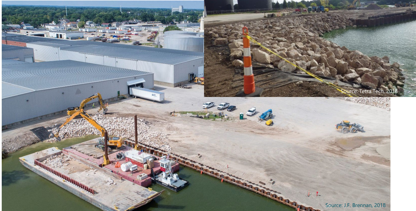
Installation of clean post-dredge buttress
