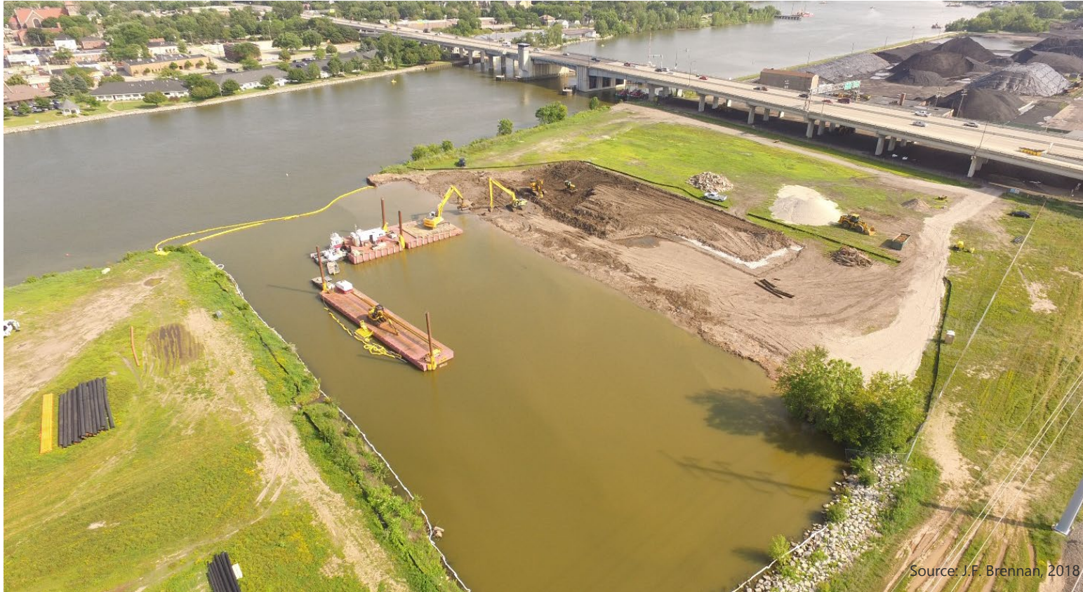
Excavation behind sheet pile walls and removal of upland surcharge load
