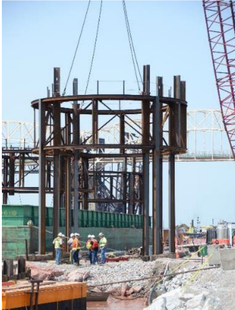
Template to be used to construct circular steel sheet pile cells
