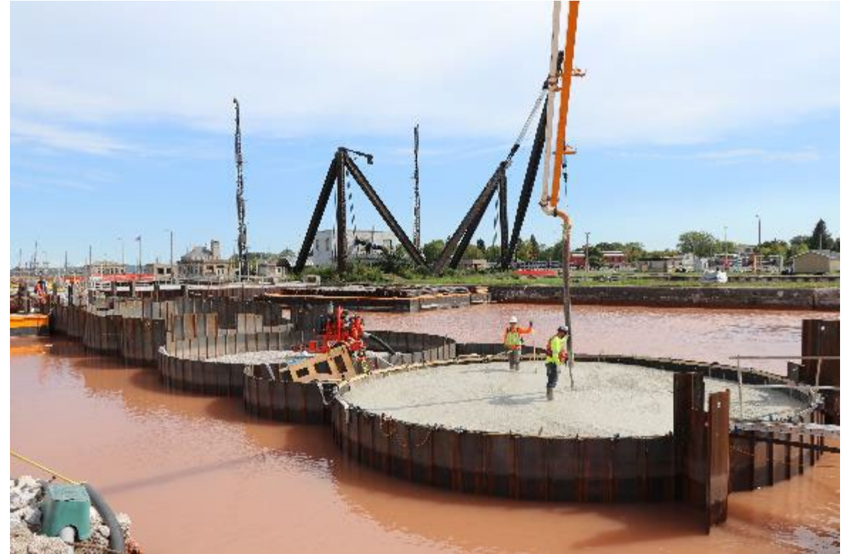
First concrete placement in cell
