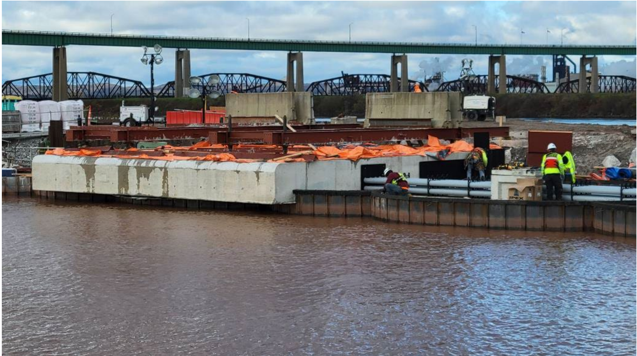
Cell SL2 Concrete Cap
