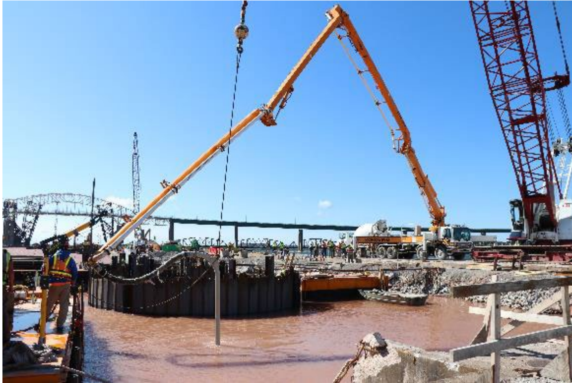
First tremie concrete placement
