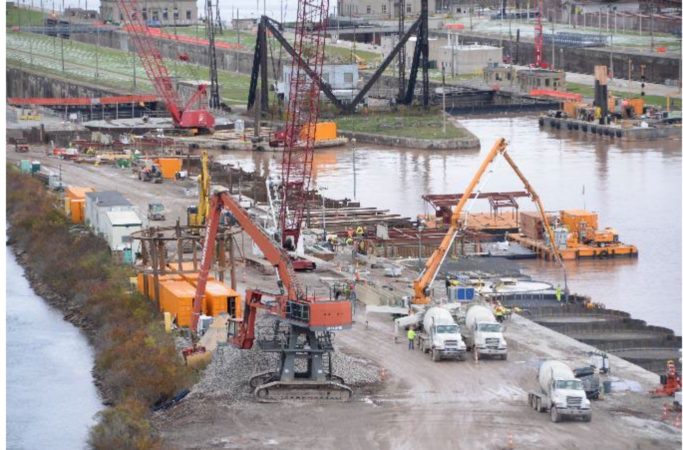
Upstream Approach Wall Tremie Concrete Placement
