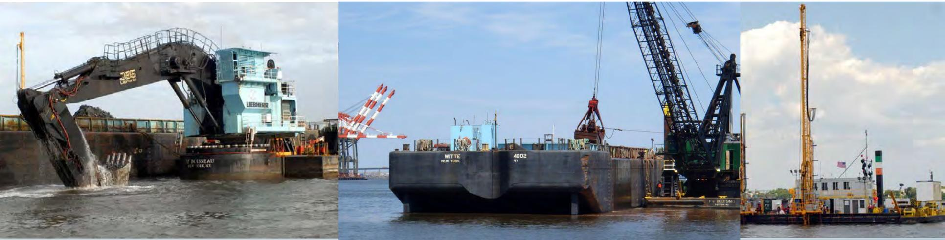
The Channel deepening effort -- part of a more extensive harbor-dredging project to create safe and efficient channels for a larger class of ships that will be calling at the Port of New York and New Jersey.
