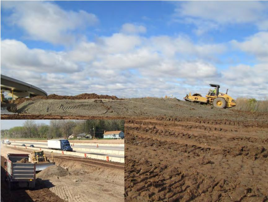
Approved sand from Lower Fox River project being used in road base construction
