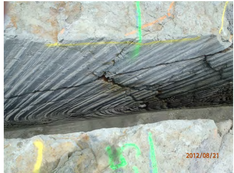
Open fractures on Dam Foundation
