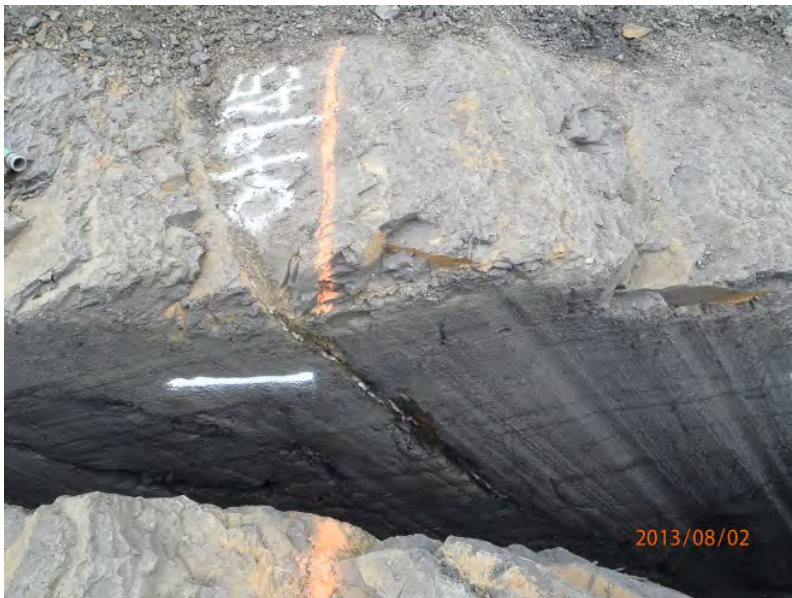
Open fractures on Dam Foundation
