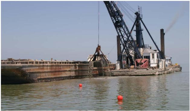
Figure 1. MCM Marine bucket dredge removing maintenance material from Maumee Bay. Red buoys marking positions of turbidity sensors shown in the foreground.
