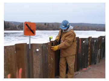
Figure 10. The integrity of the sheet pile wall is monitored by the CQA/environmental monitoring engineer due to soft underlying sediments.
