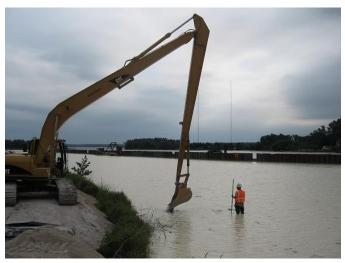
Figure 6. An alternative shoreline cap placement method, approved by the CQA/environmental monitoring engineer, included placement of uniform lifts by the RAC using a long-stick excavator.
