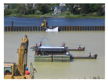
Figure 7. Activated carbon mat (ACM) was installed by the RAC after the first sand cap lift, based on the CQA/environmental monitoring engineer's cap design.
