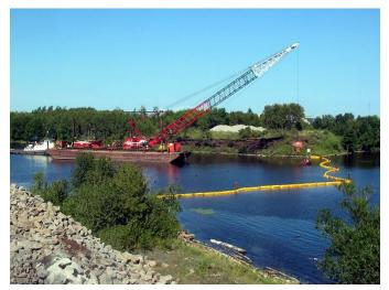
Figure 2. A crane barge with on-board GPS capabilities was used to install the pipe piles – and subsequently to place rock and gravel, which comprised the CAD end dike.
