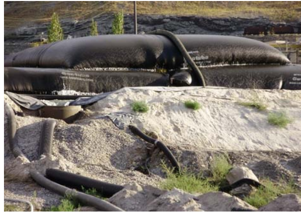
Figure 8. Lagoon near the end of dredging operations (left). Geotextile containers were stacked to minimize the space requirement for containment and dewatering (right).
