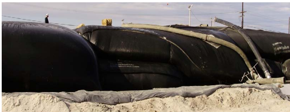
Figure 6. Geotextile containers were filled to the maximum height of 2.3 m (7.5 ft).
