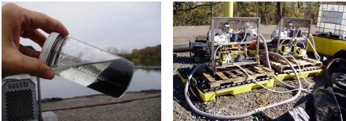
Figure 10. Lagoon residual conditioned with Solve 9248 at the project site (left). Two WSLP-2400 polymer make-down units used to deliver 20 to 30-gph of Solve 9248 (right).
