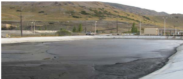
Figure 4. Full lagoon prior to commencement of dredging operations.
