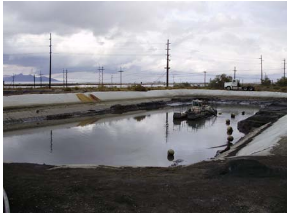
Figure 8. Lagoon near the end of dredging operations (left). Geotextile containers were stacked to minimize the space requirement for containment and dewatering (right).
