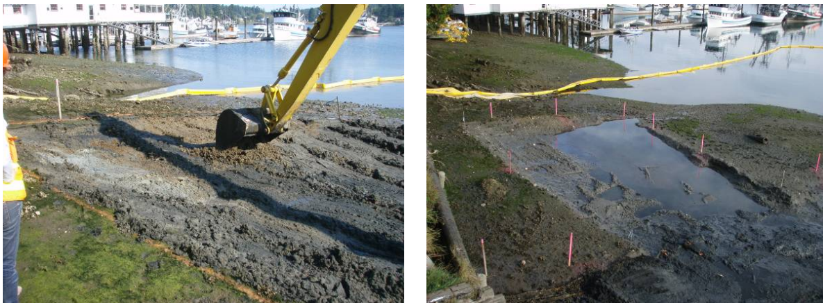
Figure 7. Dredging with long-reach trackhoe, with area delineated using survey stakes.
