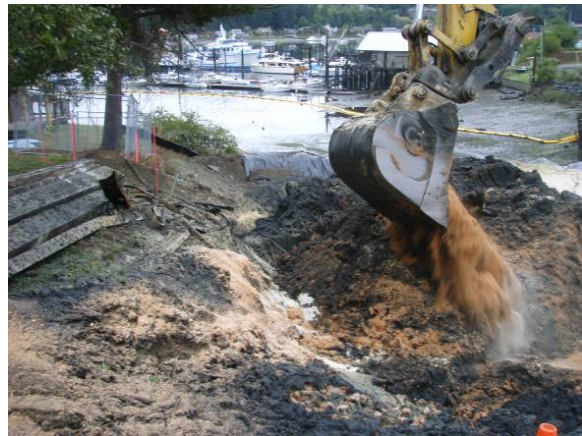
Figure 9. Mixing of sawdust and diatomaceous earth into sediment to promote dewatering.
