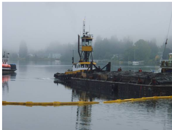
Figure 10. Removal of dredged sediments by barge.
