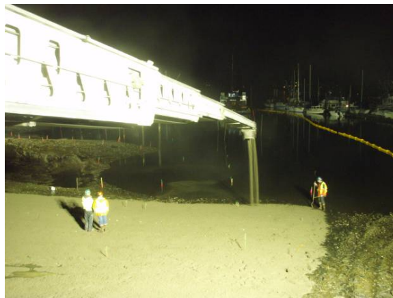
Figure 12. Placement of sand cap using a telescoping conveyor belt.
