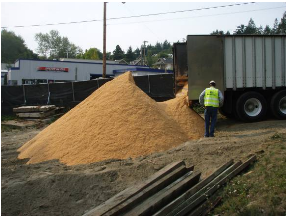
Figure 9. Mixing of sawdust and diatomaceous earth into sediment to promote dewatering.
