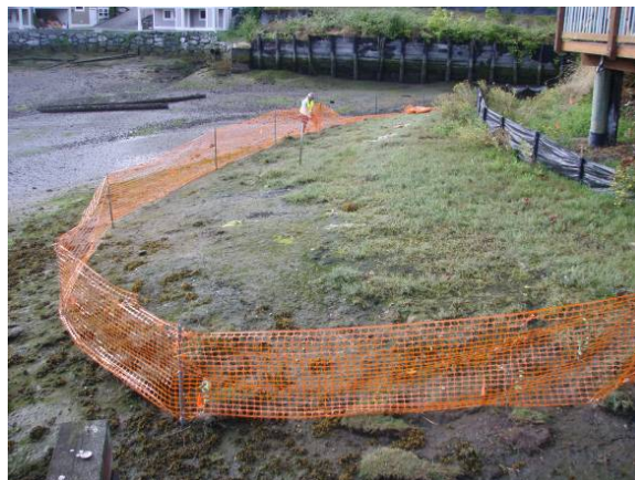
Figure 15. Installation of high-visibility construction fencing around saltmarsh vegetation area.
