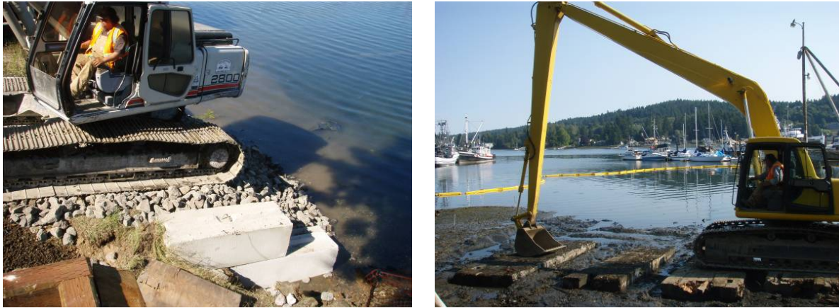
Figure 6. Use of gravel ramp and log mats to provide access for land-based dredging equipment.
