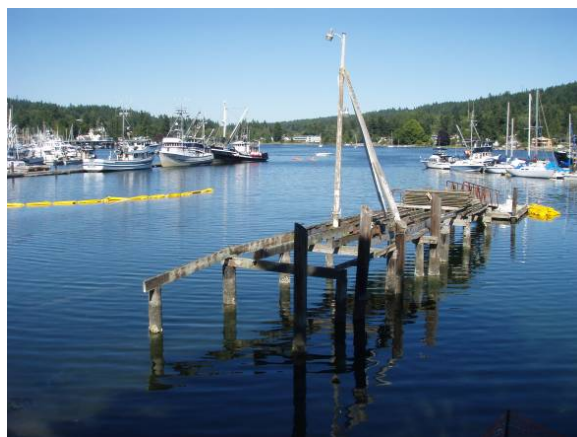
Figure 3. Timber pier structure to be removed prior to dredging.
