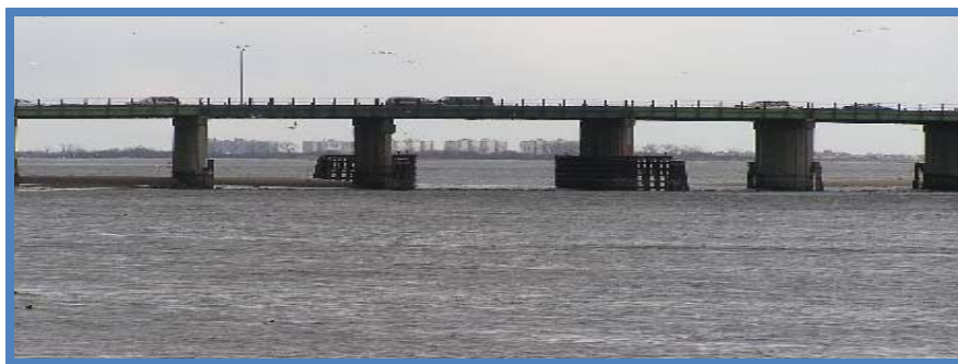
Figure 10. Belt Parkway bridge over Paerdegat Basin.
