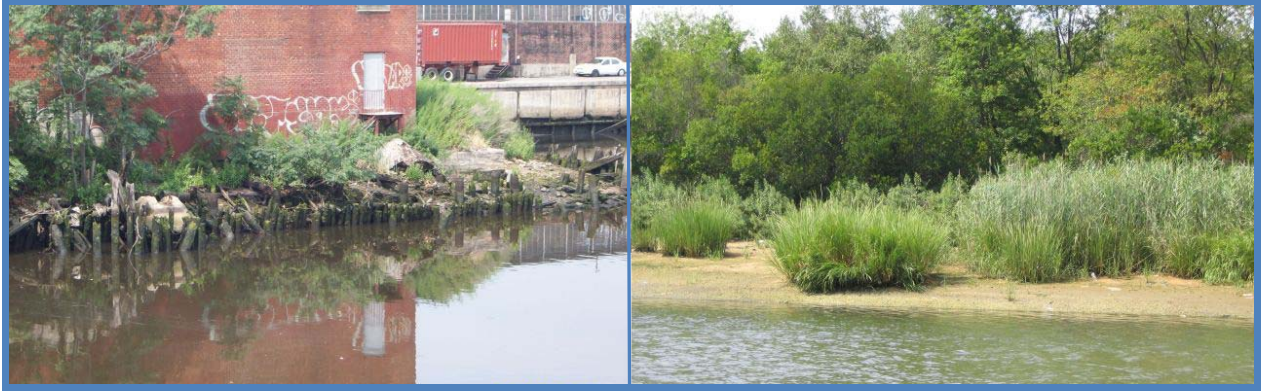
Figure 4. Undermining vegetation and structures should usually be prevented in near-shore dredging.
