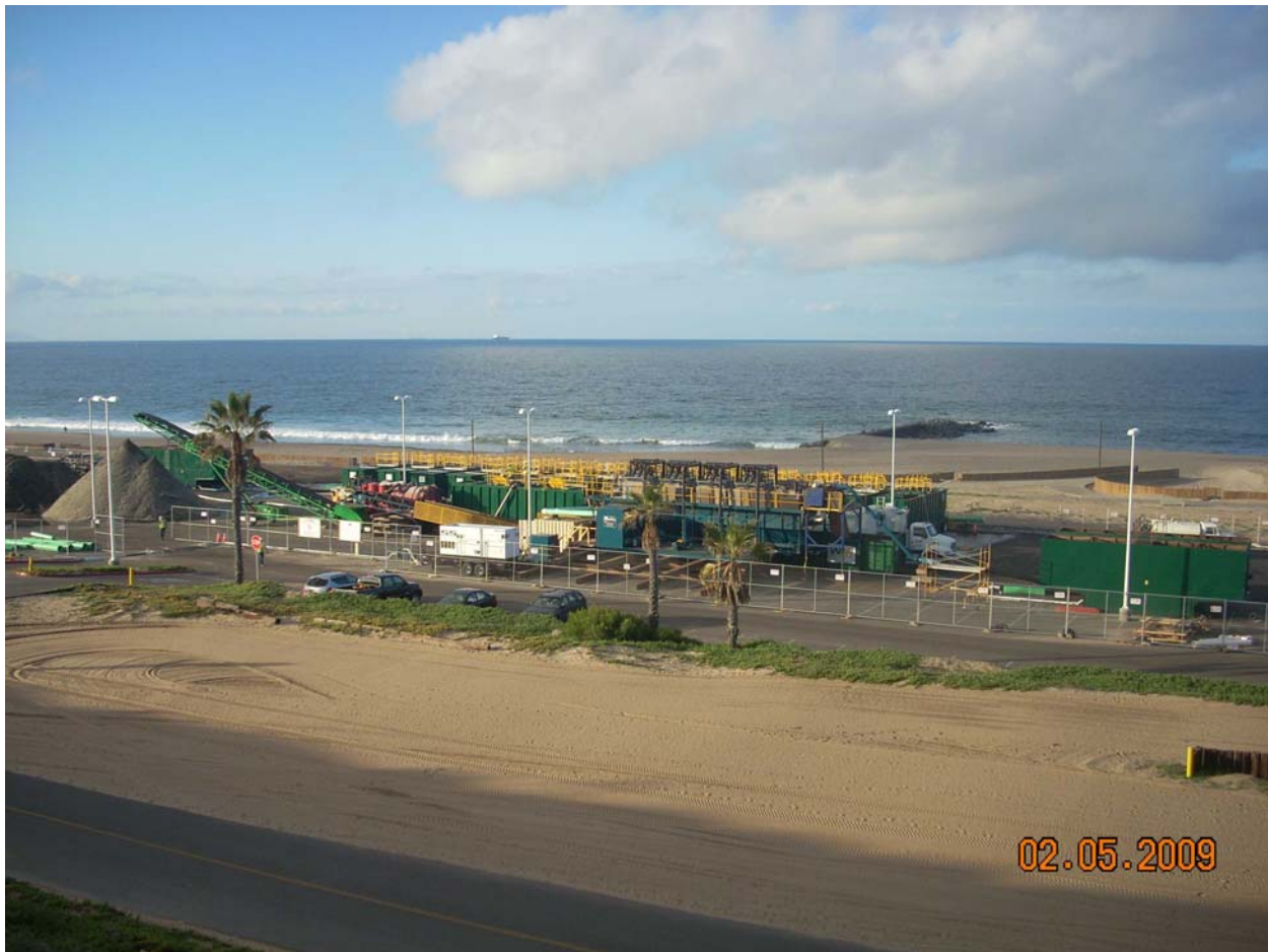
Figure 5. Operational Physical Separation System at Dockweiler Beach
