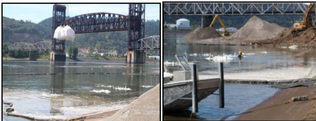
Figure 6. Placement of granular organoclay (2004).
