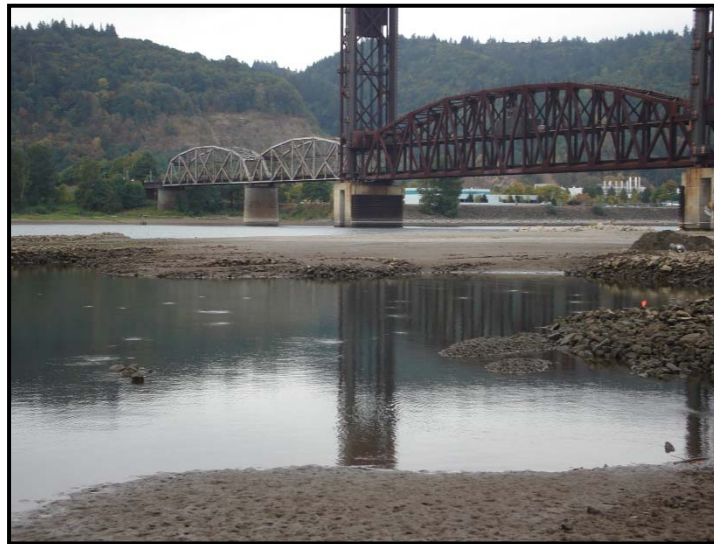
Figure 5. Ebullition in the former Tank Farm Area (2006).
