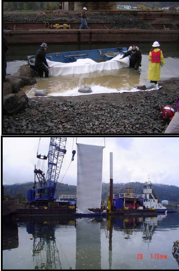
Figure 10. Organoclay Reactive Core Mat® placement under the BNR bridge (2005).
