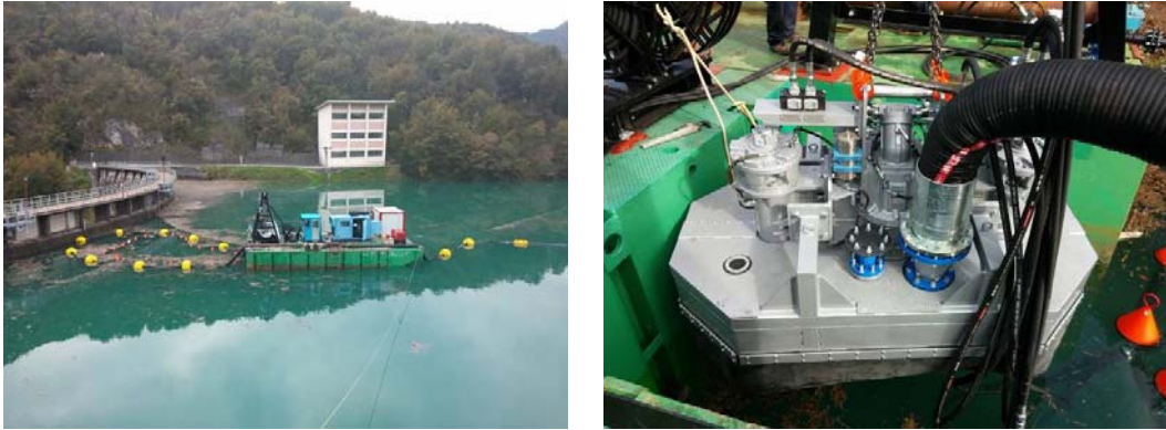
Figure 1 and 2. Dam cleaning project.
