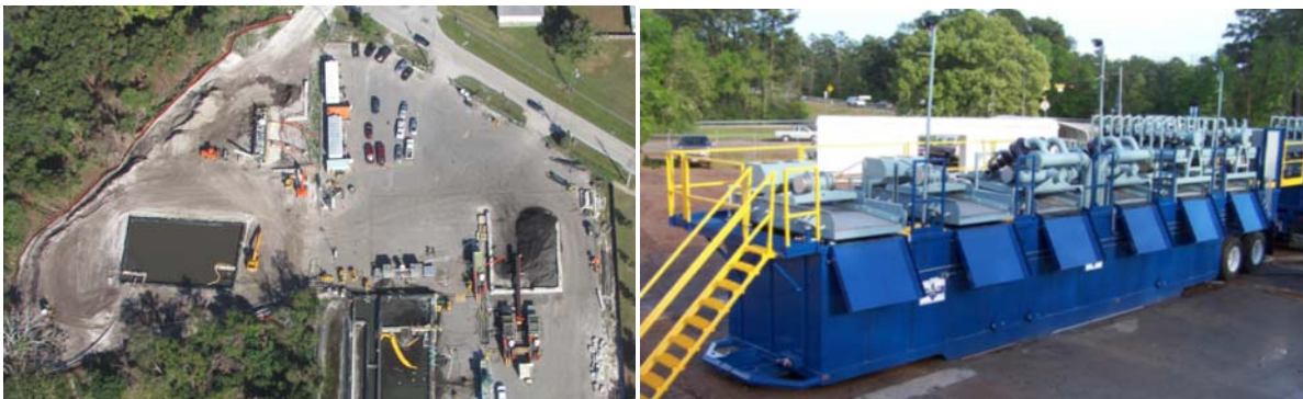
Figure 4. Overbrook Ave. dewatering site and DSS2000 Tri-Flo.
