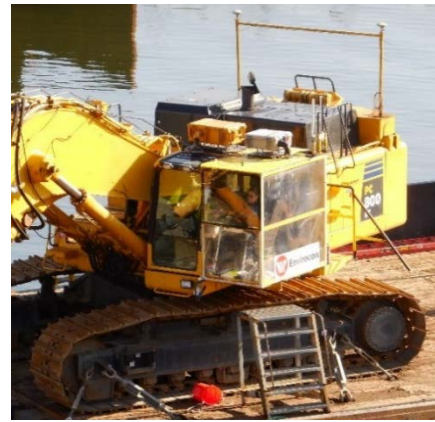
Photo 14 – Engineer in cab working with operator provides efficient, focused operation.
