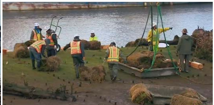
Photo 12 – Installation of pre-vegetated mats in habitat area.
