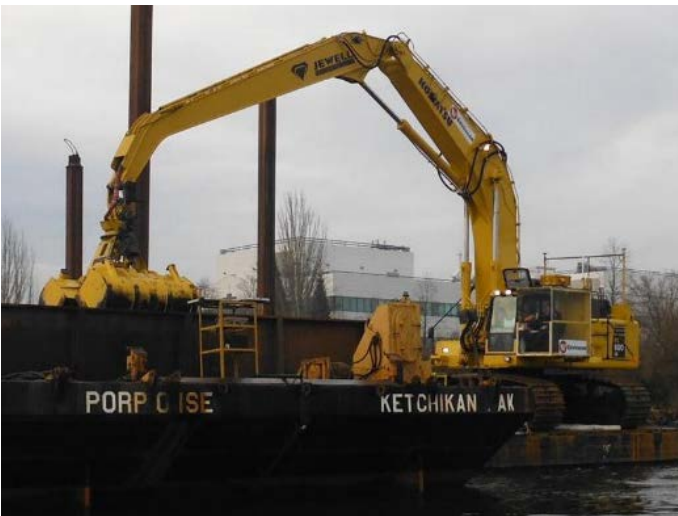
Photo 15 – Precision instrumented fixed arm excavator dredge provides needed accuracy.
