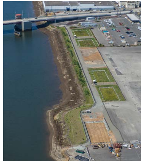
Photo 4 – South Habitat Area
