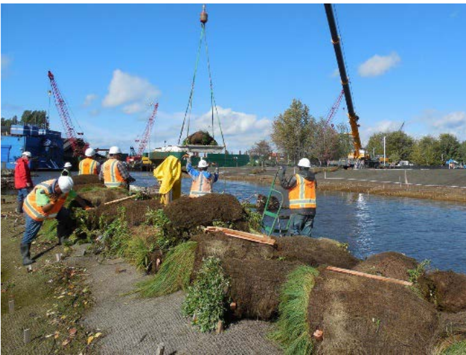
Photo 9 – Installing Native Plants using pre-vegetated mats
