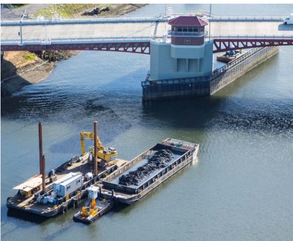
Photo 5 – Dredging of the waterway to remove contaminated sediment and restore intertidal habitat.
