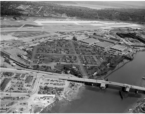
Photo 1 – A 26-acre make-believe village was constructed on top of Plant 2 to provide wartime cover. The Army Corps of Engineers dismantled the canvas cottages, wire mesh trees, and burlap lawns in 1946.
