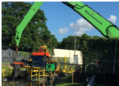
Sennebogen Removing Debris and Dredging in Wagner Creek
