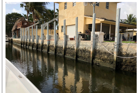
Seybold Canal Residential Seawall
