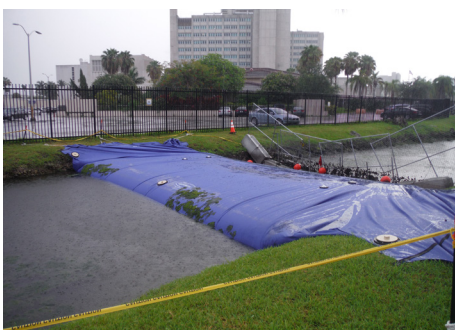
Manatee Exclusion Aqua Dam in Wagner Creek
