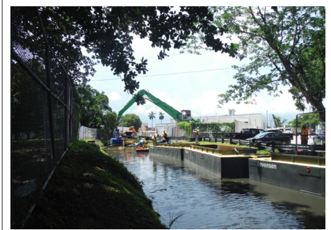
Environmental Clamshell Sennebogen and Sediment Scows
