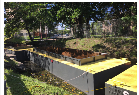
Sediment Scows Dredging in Wagner Creek
