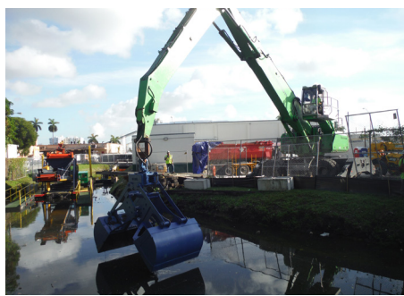
Environmental Clamshell and Sennebogen Dredging in Wagner Creek
