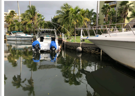
Seybold Canal Seawall
