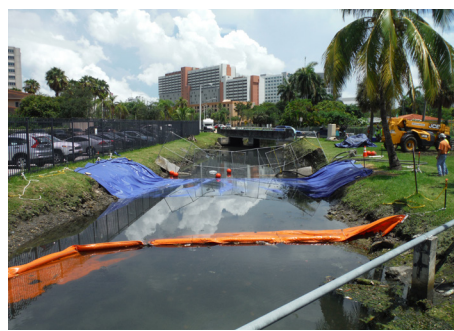
Manatee Exclusion Gates and Aqua Dam in Wagner Creek
