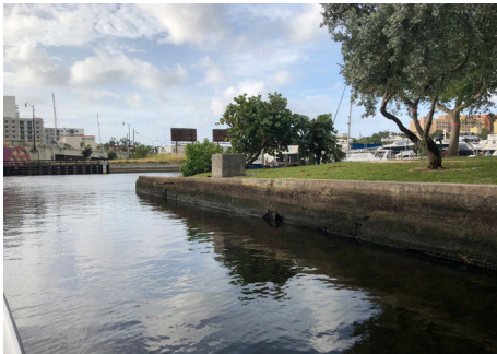
Seybold Canal and Wagner Creek Seawall
