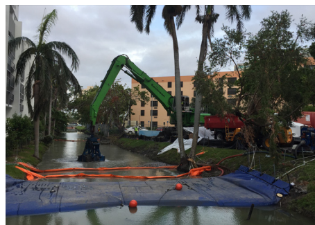
Environmental Clamshell Turbidity Barrier and Aqua Sam in Wagner Creek
