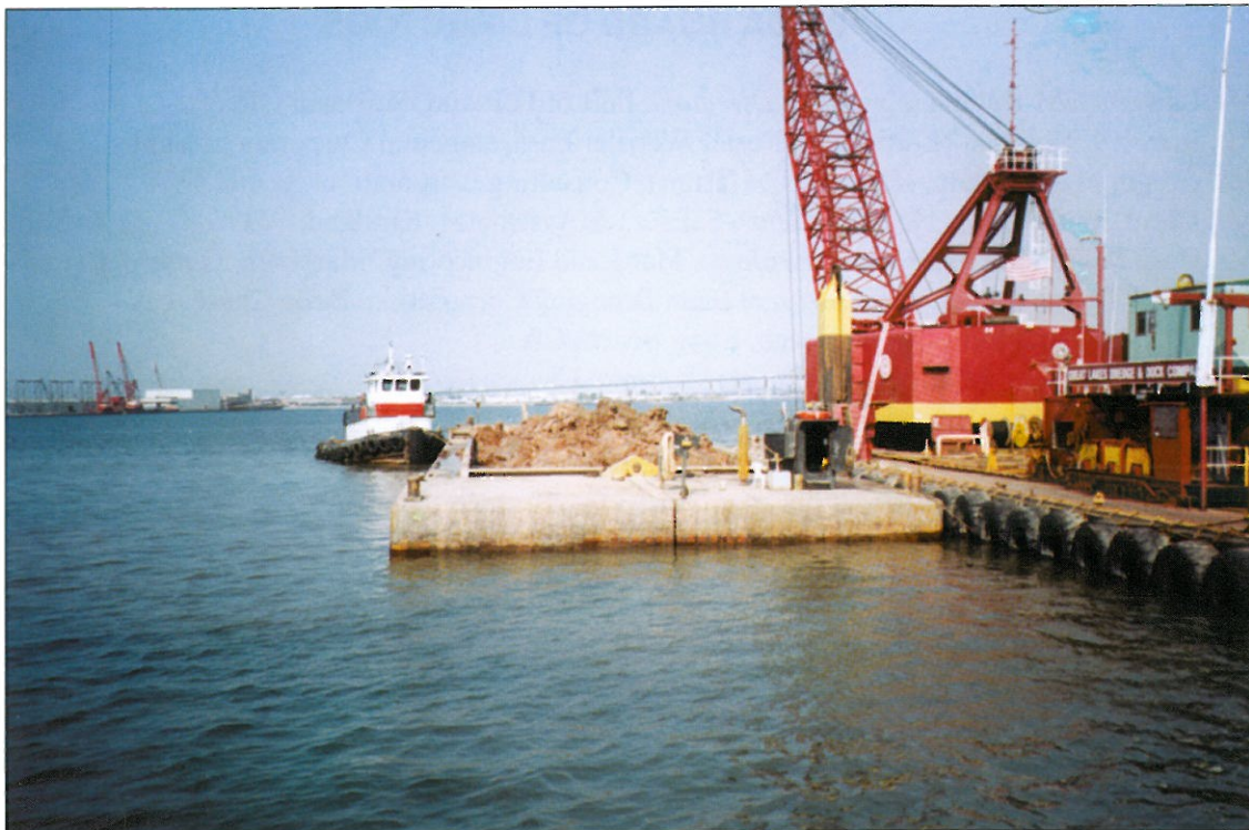
Great Lakes Dredge working in Newark Bay.
