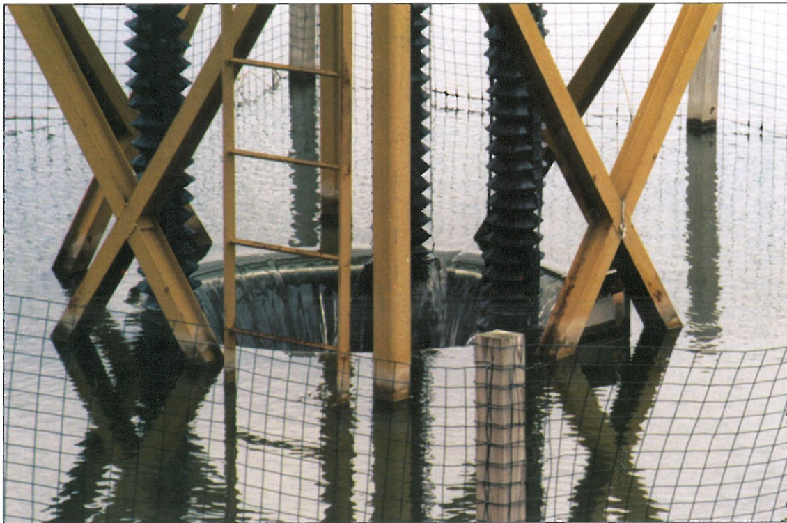
Telescoping Weir (photo courtesy of J. Fowler)
