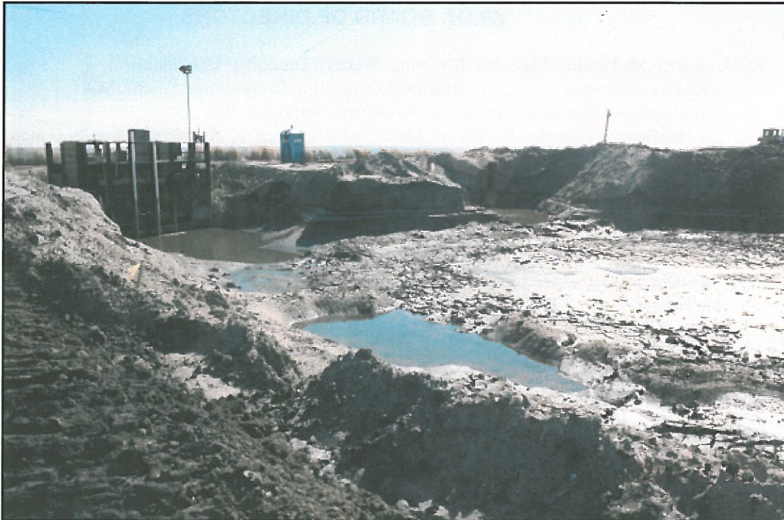
View of a Spillway at a Placement Site
