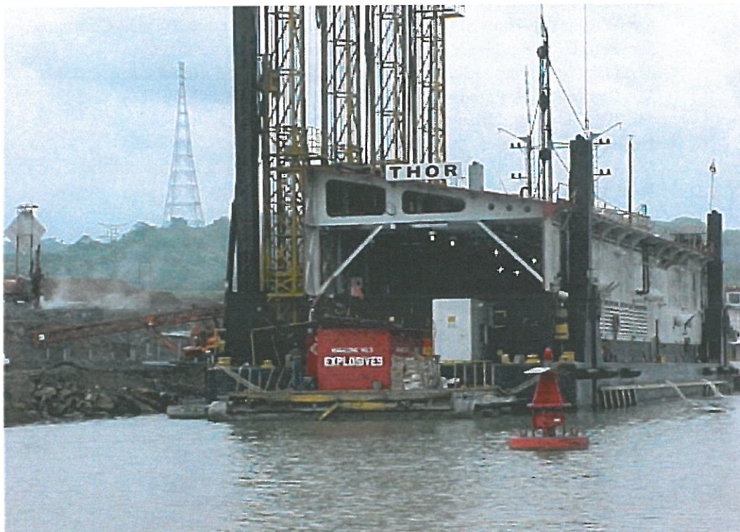
Dredge Thor in Panama Canal
