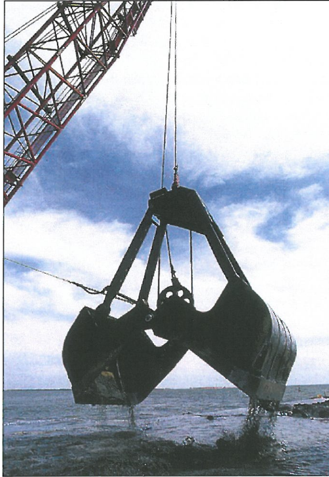
Figure 1: The 50 cubic yard clamshell buckets
