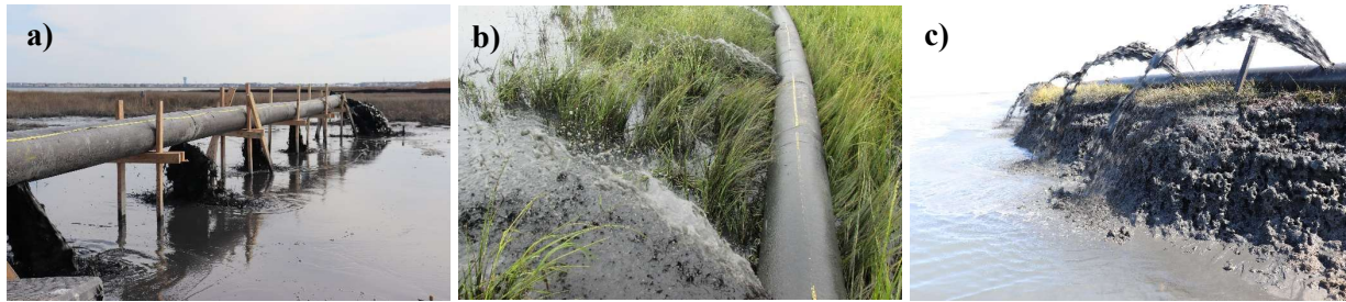
Figure 7. SDP application scenarios: (a) elevated pipe, (b) placed on the marsh surface, and (c) placed on the marsh edge to build an edge protection feature.
