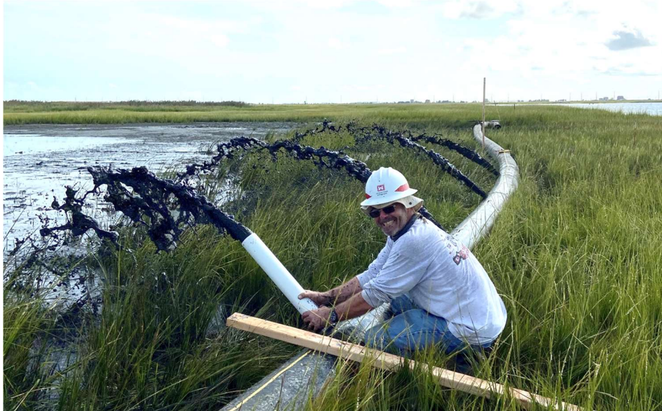
Figure 12. The late Tim Welp testing risers on the Sediment Distribution Pipe.
