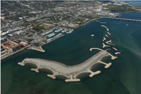
New Island Construction
